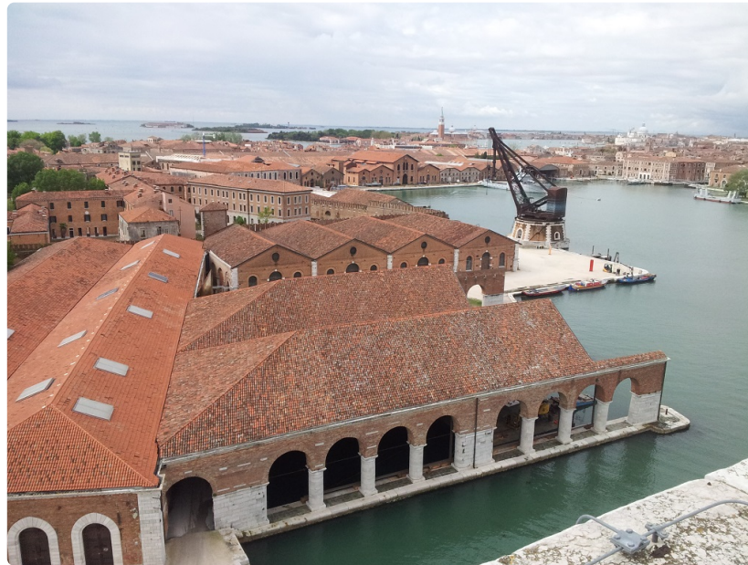
Overview of the Arsenale. Photo by Andrea Avezzù.
